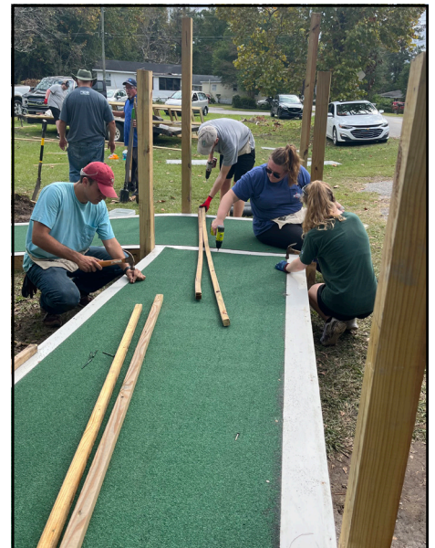
MSN builds handicapped ramp during spring break.
